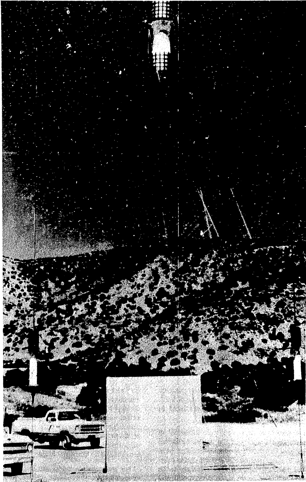
Figure 3. Bottom end drop height and orientation check (85-346-3-7).
